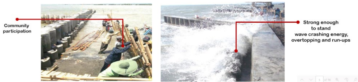
Picture 1. Groyne construction in Semarang
